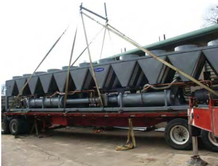
Figure 2. Delivery of 500 ton chiller
